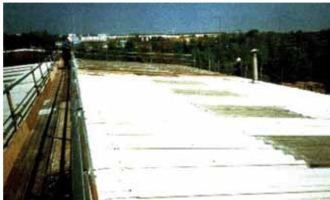
*Figure 9.5: Cleaning a fibre cement roof using a self-contained water fed brush unit. There is no need for access onto the roof sheets and the guard-rails prevent workers falling onto them. (Note: waste\water is filtered before disposal).*
