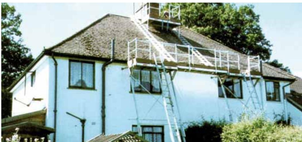
*Figure 8.10: Proprietary system for access to roof and chimney.*
