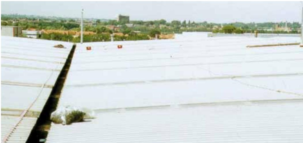
*Figure 9.6: In some light conditions it is difficult to distinguish the rooflights from the metal sheets on this type of roof. Also the valley gutter is very narrow and rooflights extend down to gutter level. Both of these features increase the risk during cleaning maintenance and refurbishment.*
