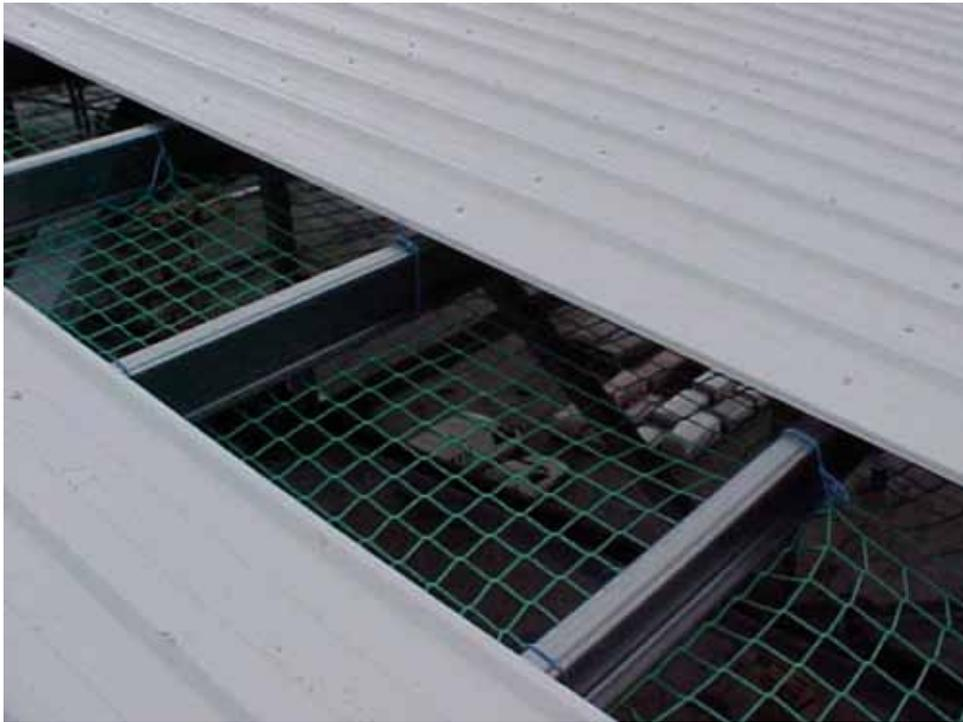
*Figure 9.3: Industrial roofwork: Use of safety nets.*
