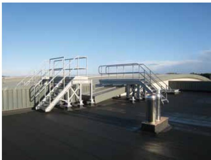
*Figure 4.2: Permanent access stairs giving safe access to different roof levels. (This permanent stair access was included in the initial design).*
