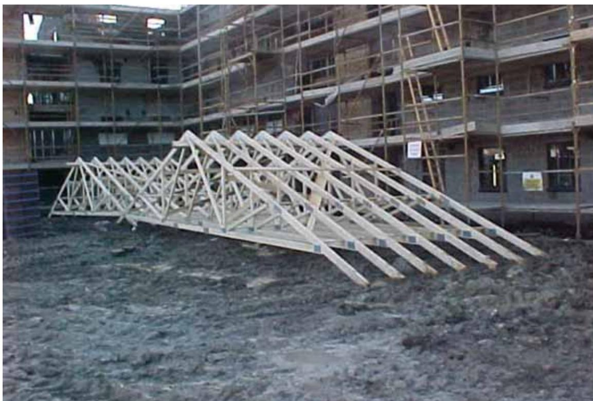
*Figure 8.1: Lifting pre-assembled roof into position by crane greatly reduces the need for work at height.*
