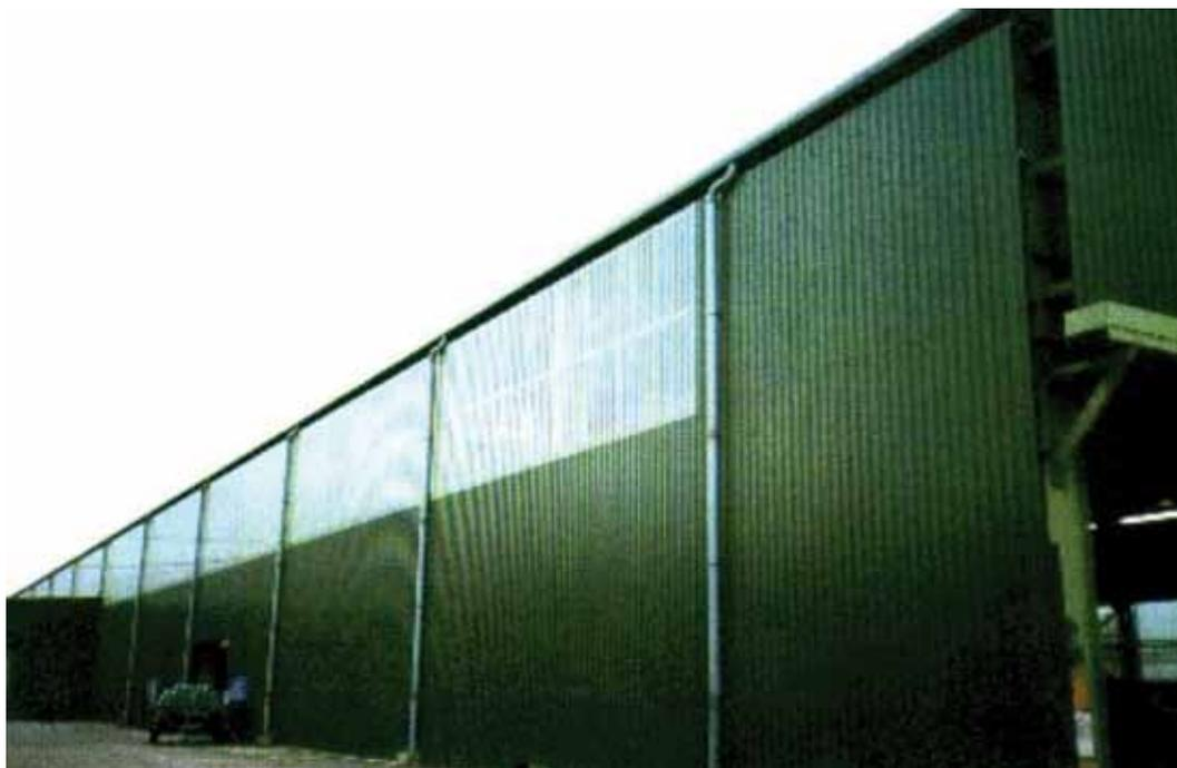
*Figure 4.3: Lighting panels installed in the walls rather than the roof.*
