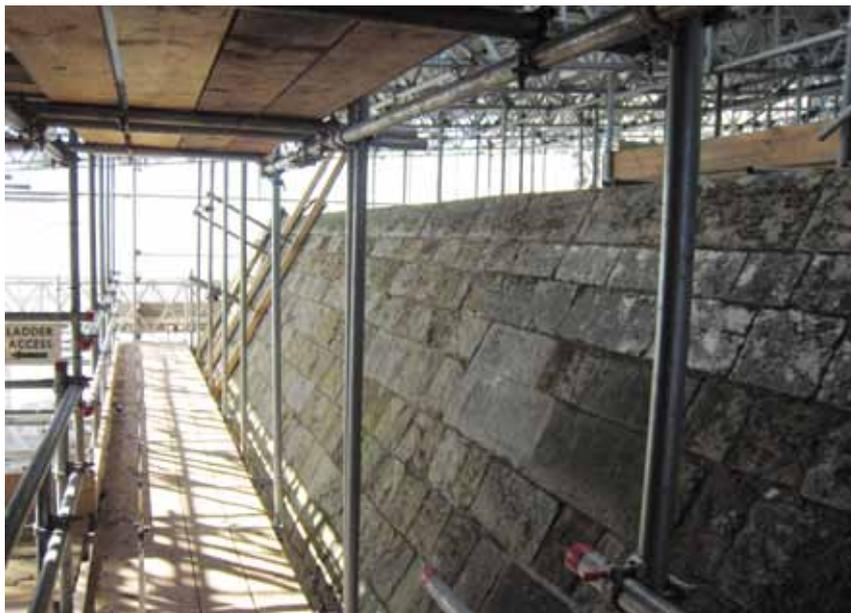
*Figure 11.1 Providing safe access and a safe working platform at roof level (source Office of Public Works, National Monuments).*
